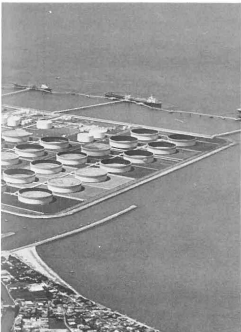
Kiire Oil Relay Terminal. This terminal has now a storage capacity for 6.6 million kilolitres.
